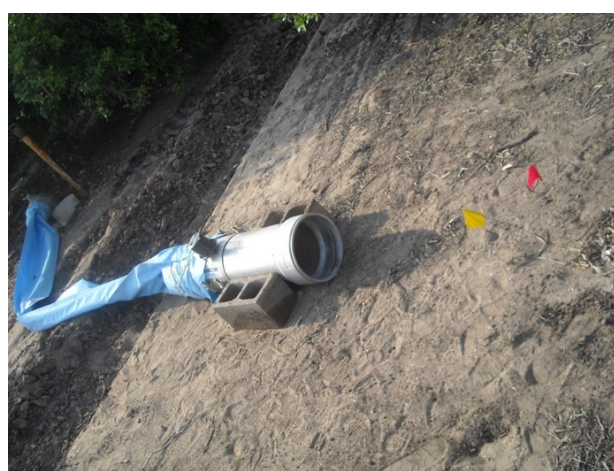
Fig. 3. Flood irrigation outlet pipe valve attached to polypipe and connected to a 30-cm dia. pipe affixed with water metering device.
